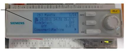
3) ADJUSTING THE OPERATING MODE – The "Protection" / "Economy" / "Comfort" / "Schedule" operating mode must be selected to start the unit Press the button for the "Comfort" operating mode for standard operation.
